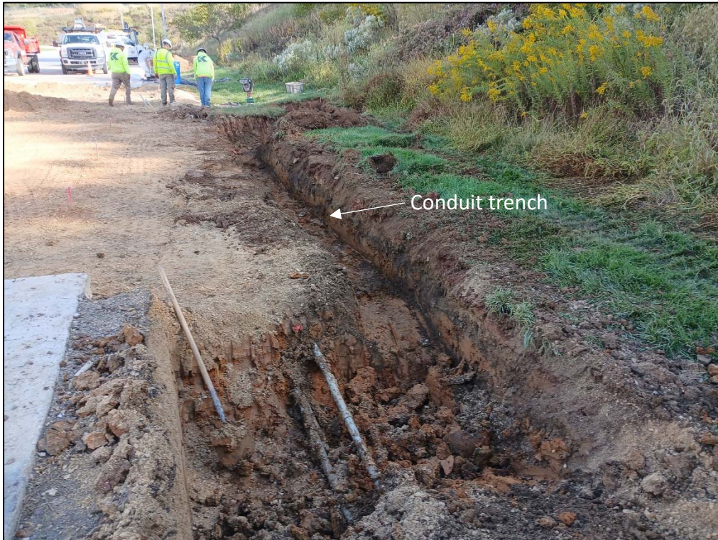
Photo 4: Photo looking north at exposed conduits south of dock replacement area and conduit trench from light pole excavation.
