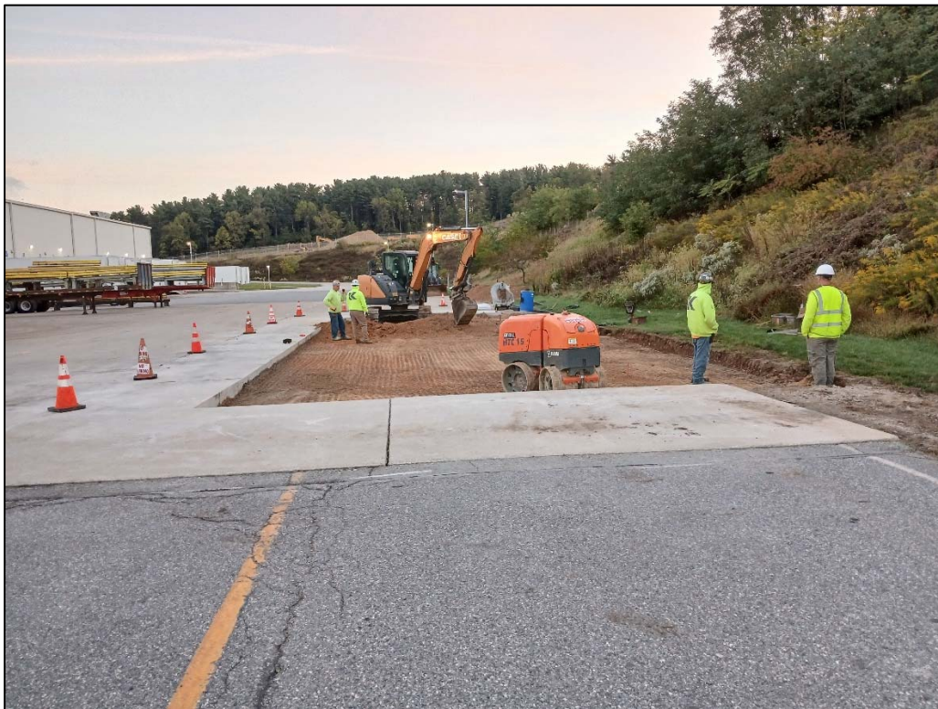
Photo 2: Concrete removed from existing dock and five foot area to the east was excavated.
