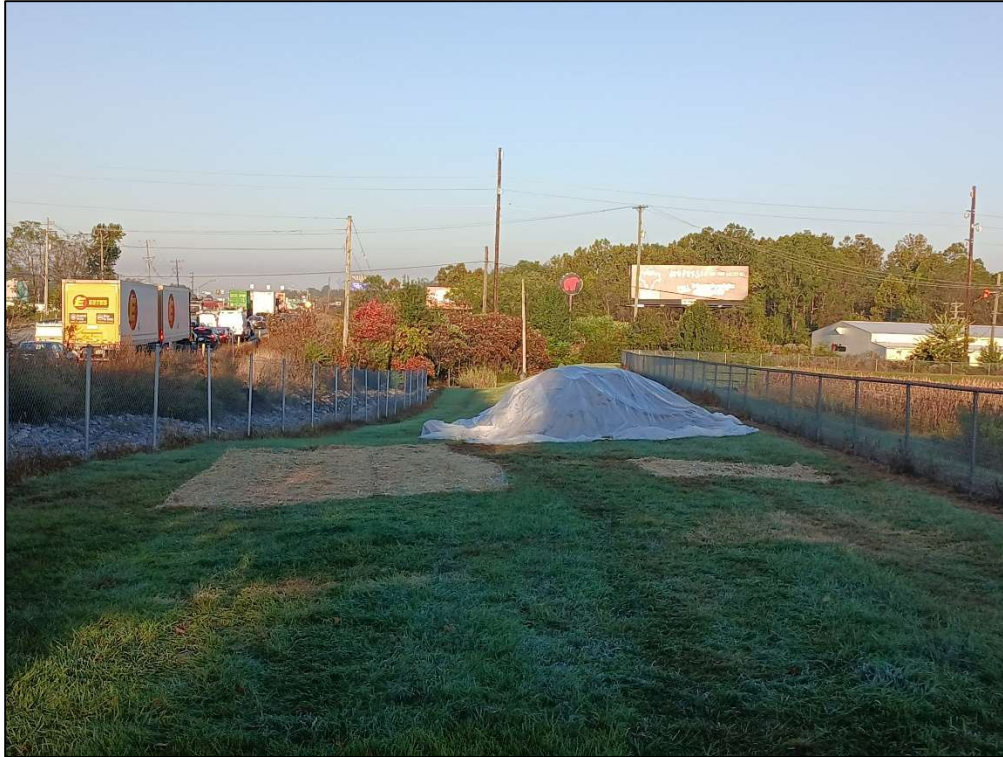
Photo 7: Sinkhole repair area was seeded, and straw matting was installed. The excavated soil stockpile is on and covered with plastic.
