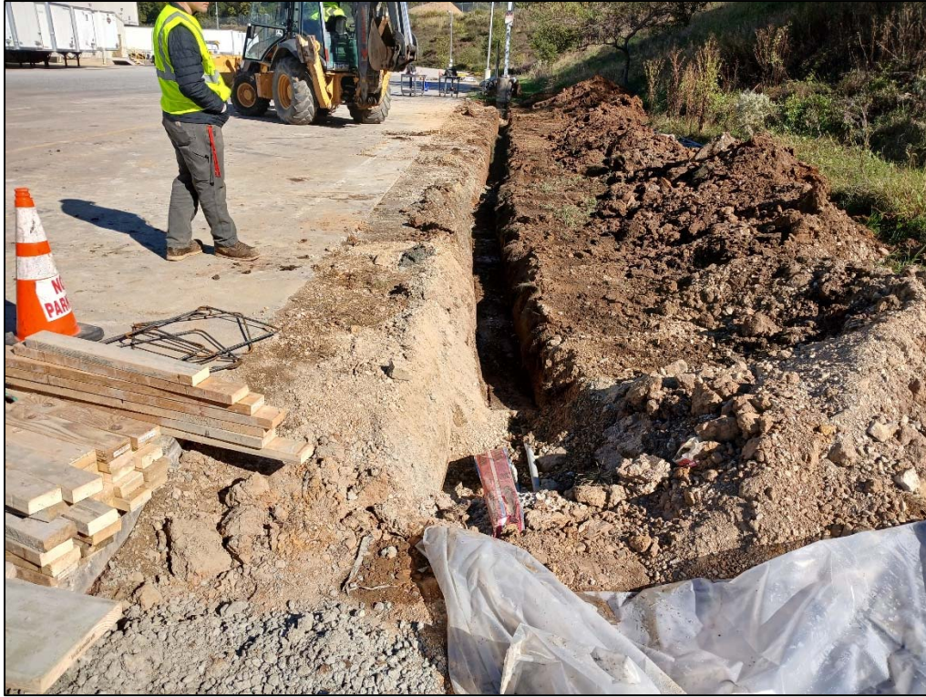
Photo 5: Photo looking north at conduit trench north of dock replacement area to the next existing light pole.
