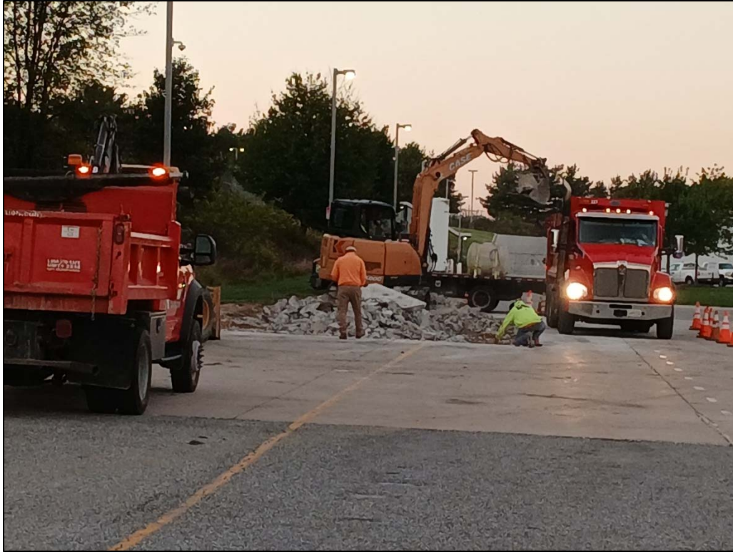
Photo 1: Kinsley removing existing dock concrete.
