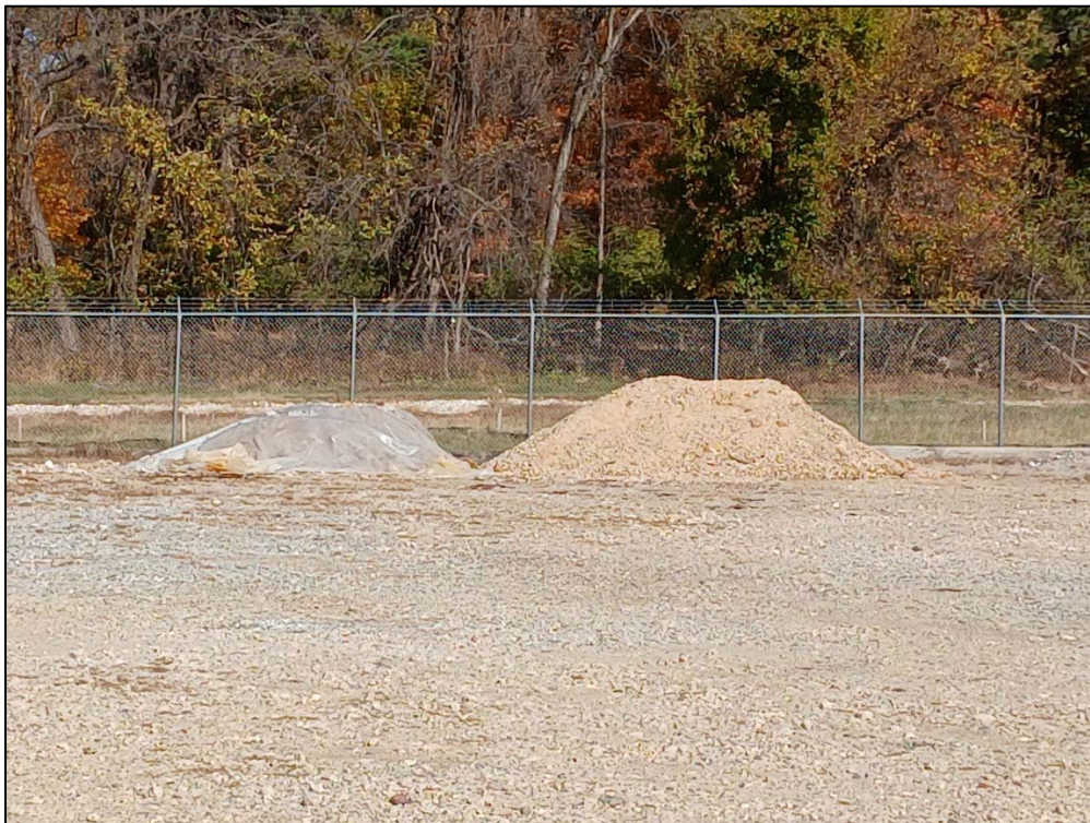
Photo 8: Excess soil is under plastic, and the excess stone is stockpiled at the north end of the contractor's lot.
