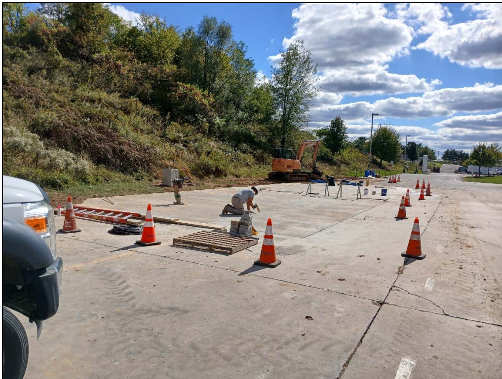
Photo 6: Photo looking south at concrete replacement area.
