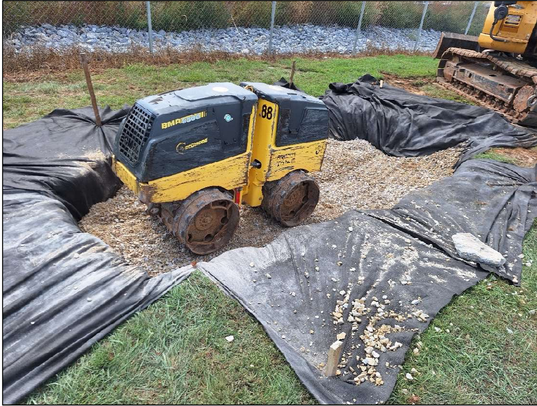
Photo 5: 2A stone installed and compacted with vibratory roller.
