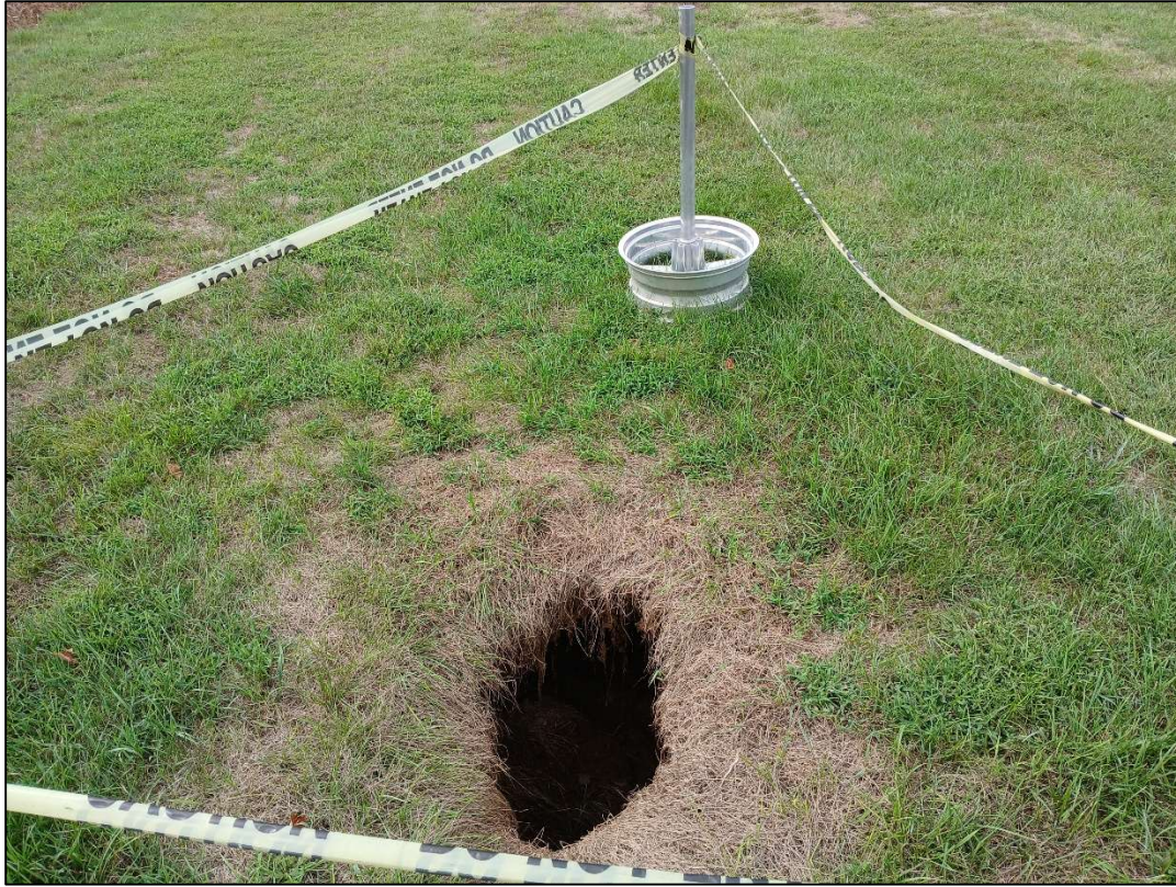
Photo 1: Sinkhole prior to repair work.
