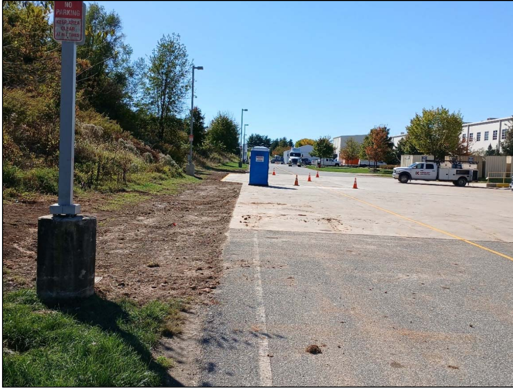
Photo 7: Photo looking south at work area after conduit trench was backfilled.
