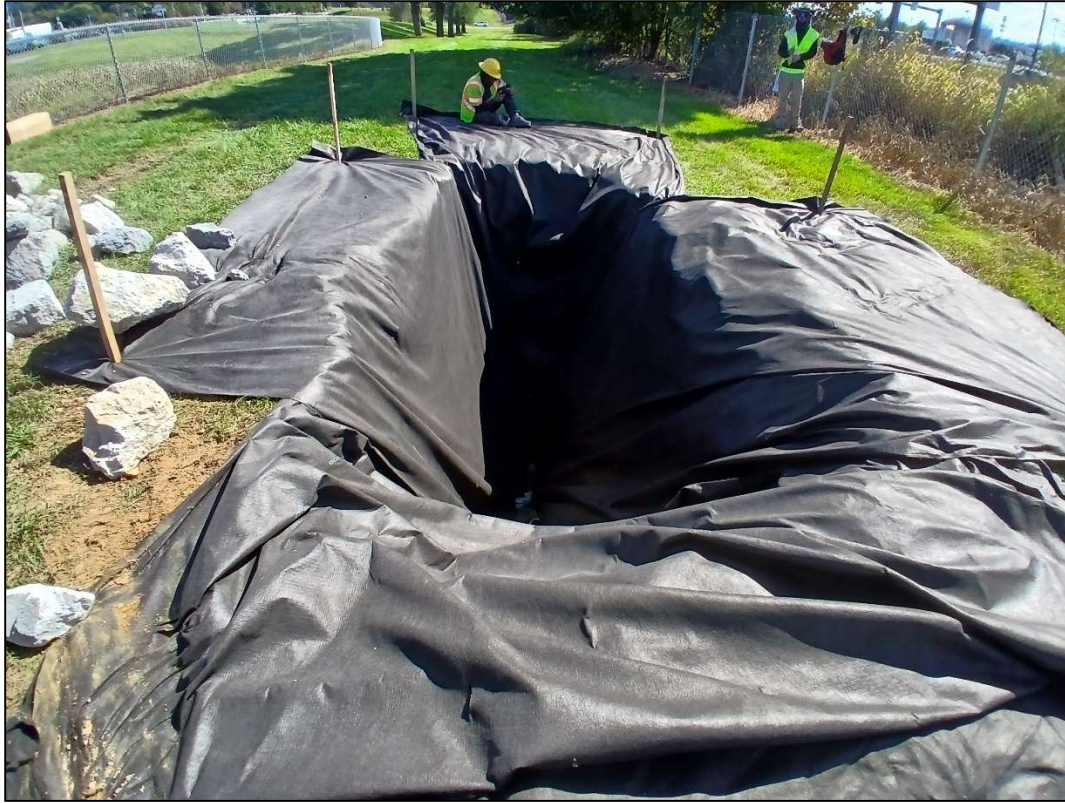
Photo 3: Geotextile fabric installed prior reverse grade stone backfill.
