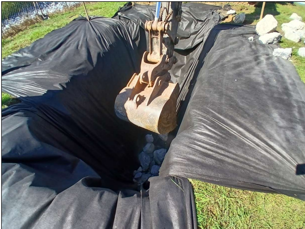
Photo 4: Begin backfill with R5 stone.
