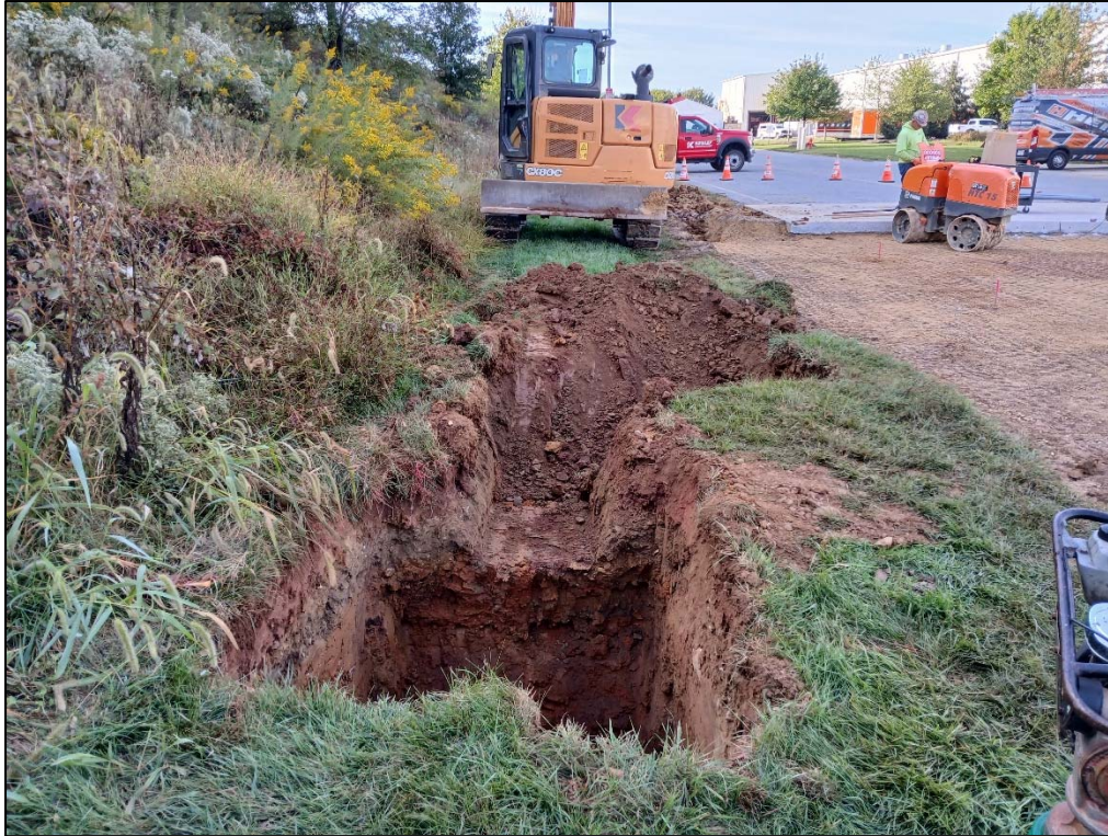
Photo 3: Photo looking south at light pole relocation excavation.
